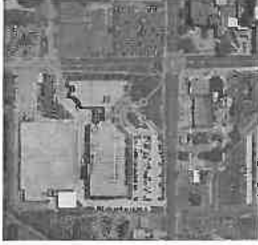
Aerial View of Existing Ambulatory Care Center
